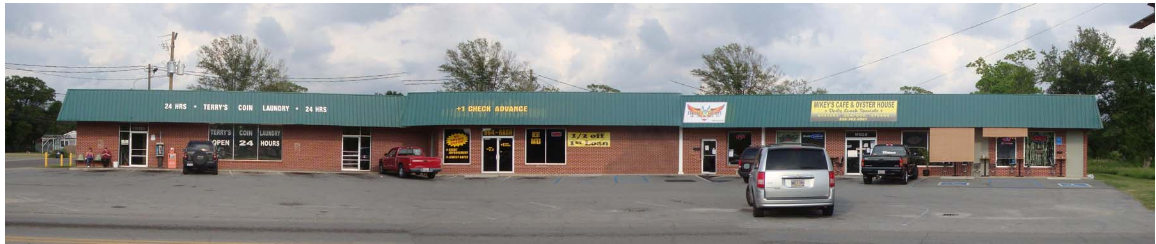
1 EXISTING FACADE CONDITION A102 NTS
