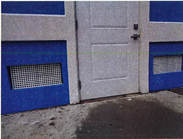
PICTURE OF TYPICAL VENT. (LENGTH VARIES) PICTURE TAKEN 03/17/2016
