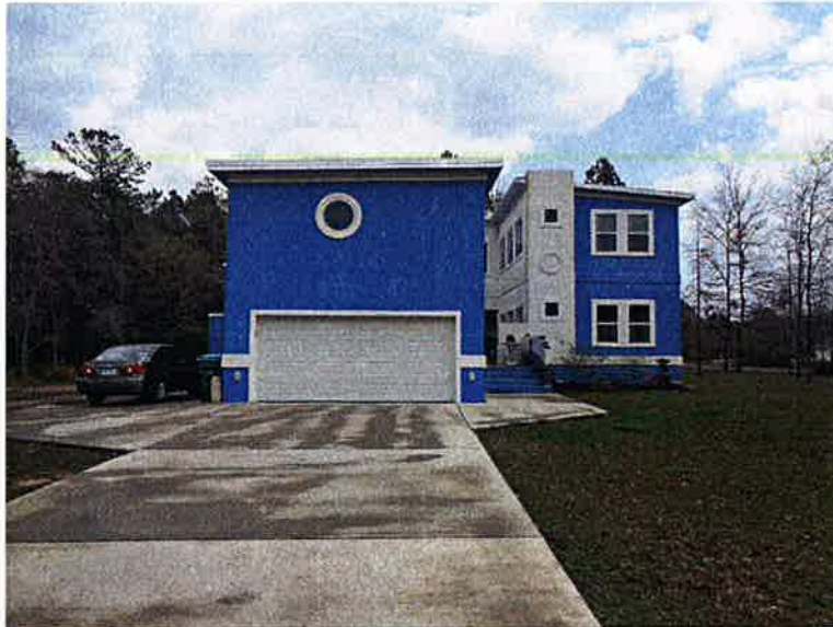
FRONT VIEW OF BUILDING. PICTURE TAKEN 03/17/2016
