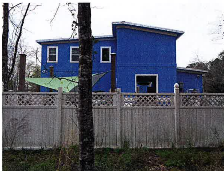
REAR VIEW OF BUILDING. PICTURE TAKEN 03/17/2016
