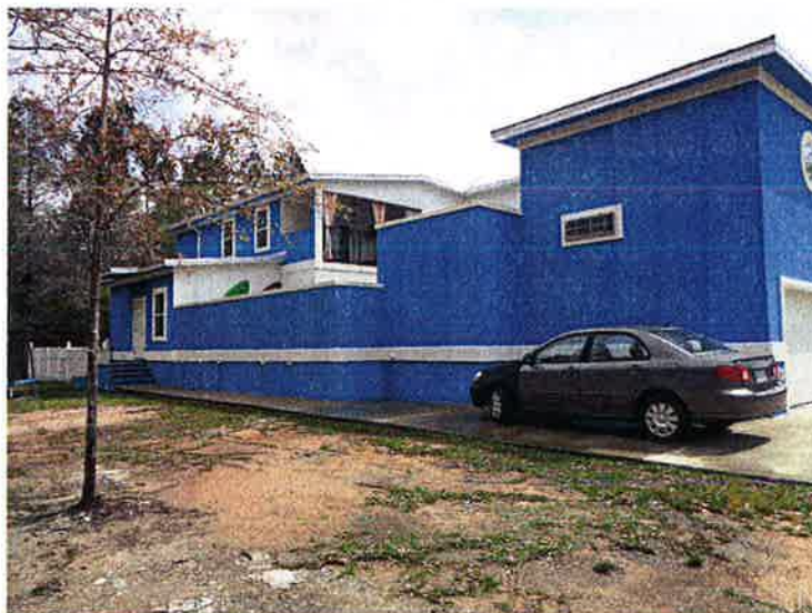
LEFT SIDE VIEW OF BUILDING. PICTURE TAKEN 03/17/2016
