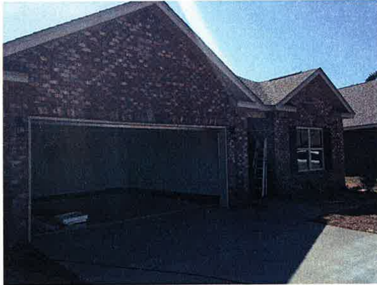
FRONT VIEW OF BUILDING. PICTURE TAKEN 03/15/2016
