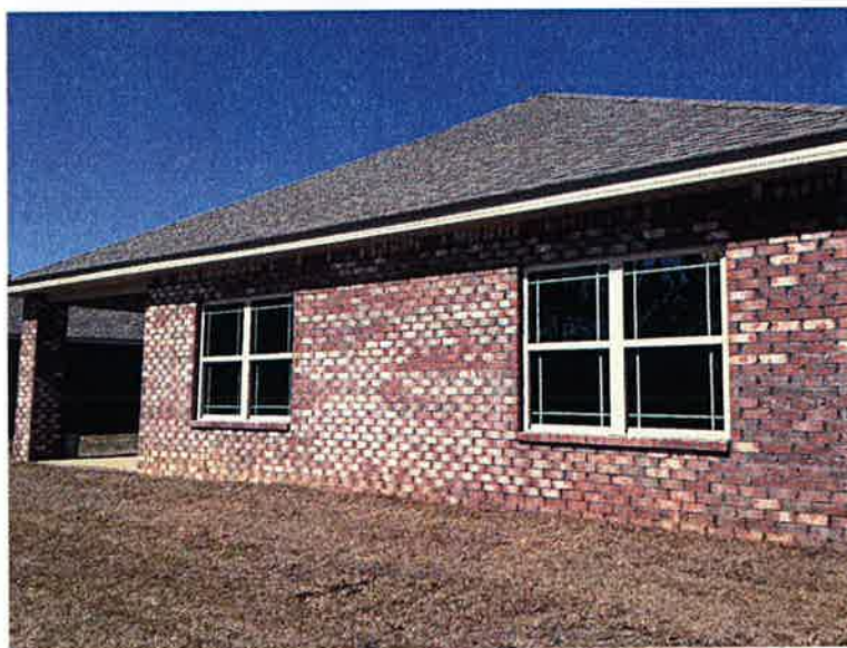
REAR VIEW OF BUILDING. PICTURE TAKEN 03/15/2016
