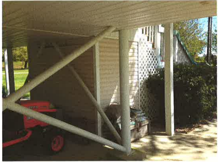
Rear view of 5'x10' enclosure under residence. 03/27/15
