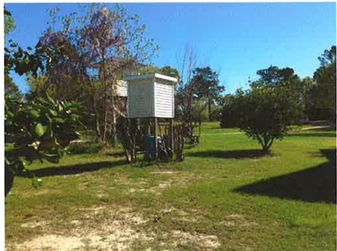
Elevated water well pump house. 03/27/15
