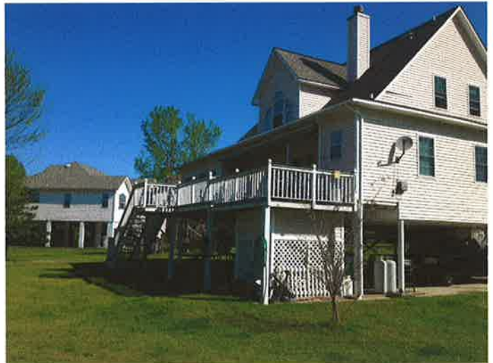
Rear view of residence, looking north. 03/27/15
