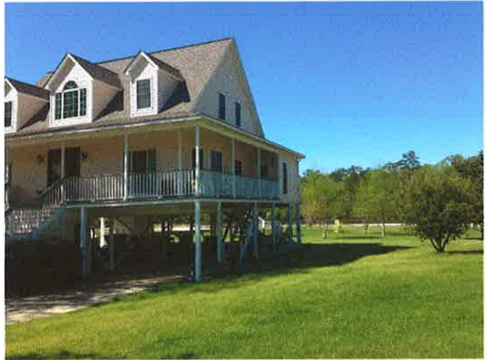
North side of residence, looking southwest. 03/27/15
