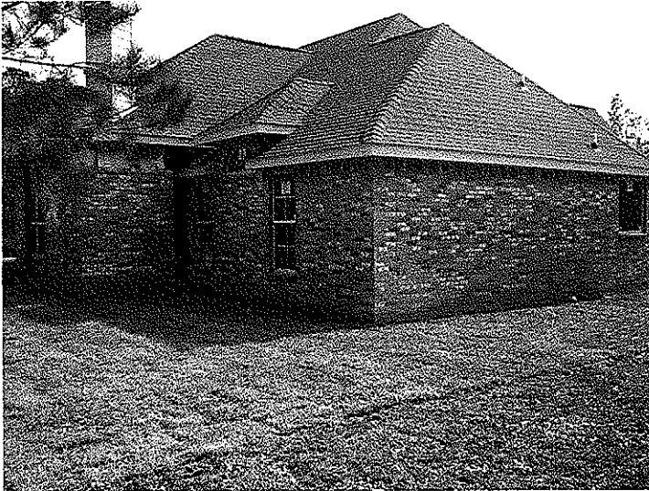
Rear left side looking Easterly.
