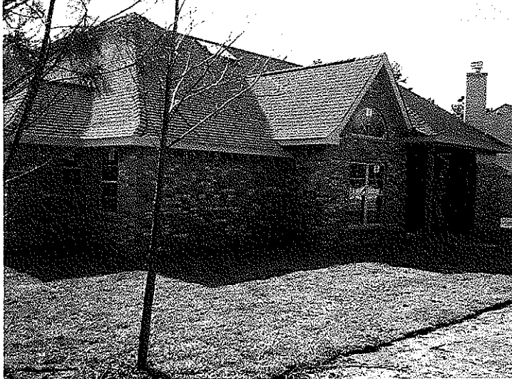
Rear left side looking Westerly.
