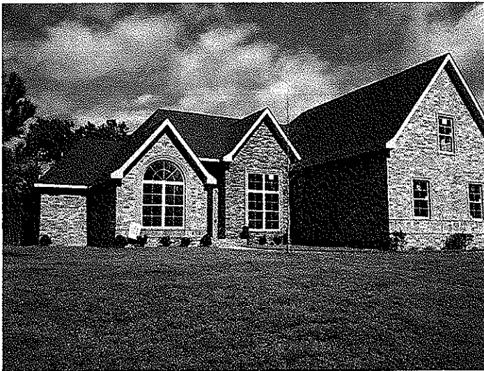
Front left side looking North.
