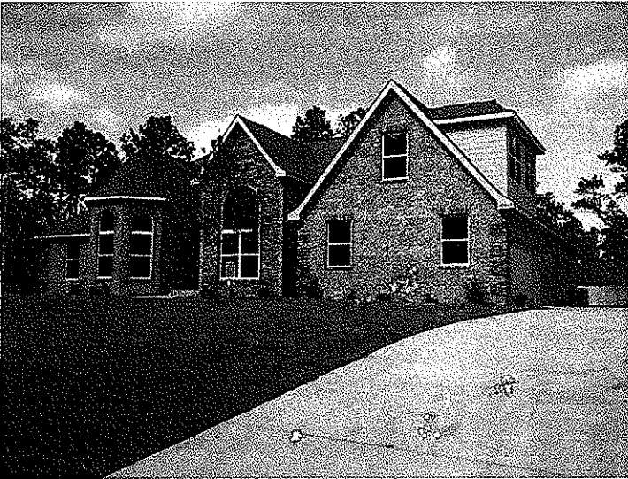
Front right side looking North.
