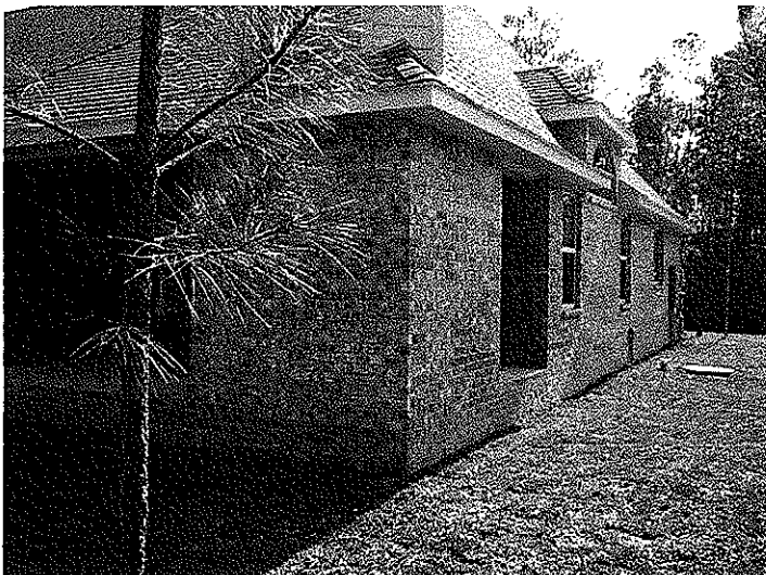
Rear left side looking Southerly.
