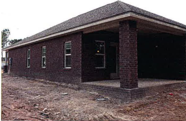
RIGHT SIDE VIEW OF BUILDING. PICTURE TAKEN 12/01/2015
