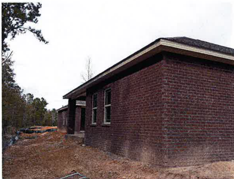
REAR VIEW OF BUILDING. PICTURE TAKEN 12/01/2015
