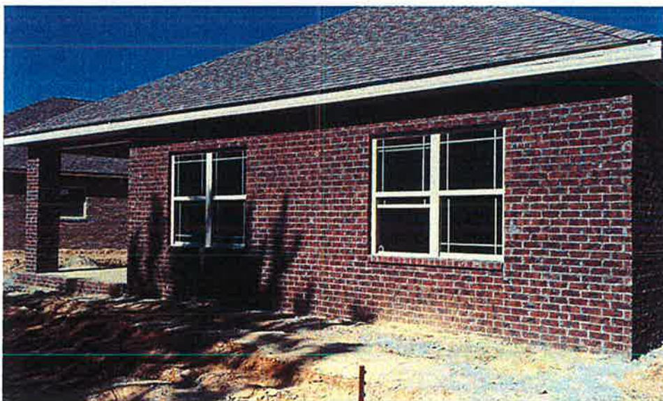
REAR VIEW OF BUILDING. PICTURE TAKEN 02/09/2016
