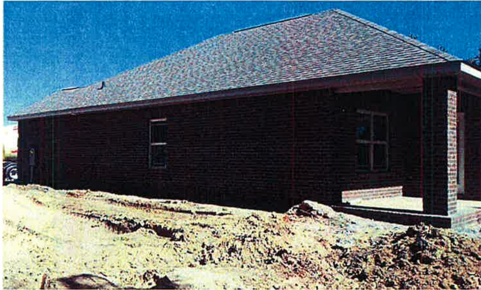
RIGHT SIDE VIEW OF BUILDING. PICTURE TAKEN 02/09/2016
