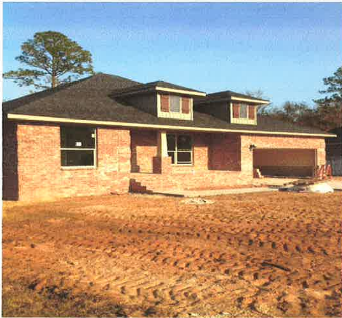
Front View Lot 25 Cypress Creek, Ph 4, looking East 12/4/12
