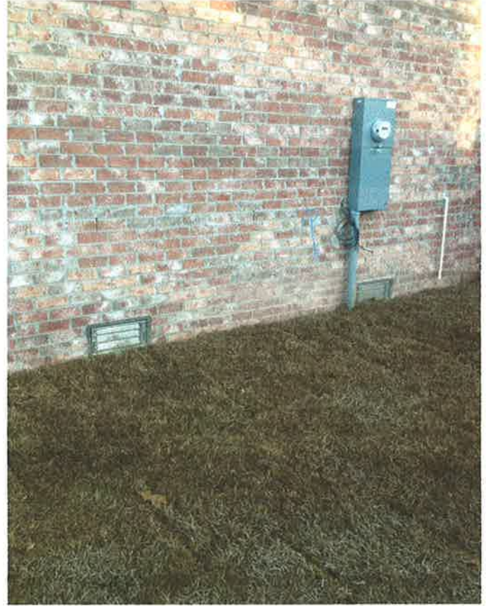
Right Side flood vents, Lot 25 Cypress Creek Ph 4, 12/13/12
