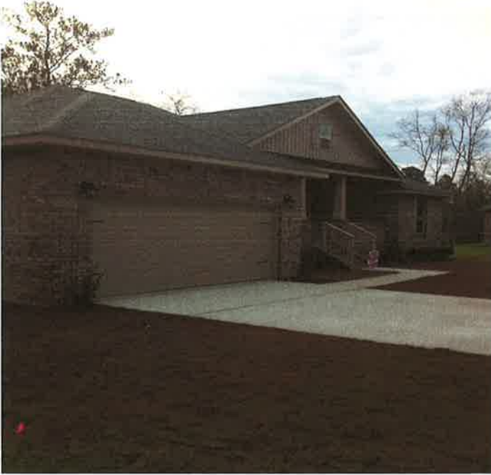
Front View Lot 26 Cypress Creek, Ph 4, looking Southeast: 2/4/13
