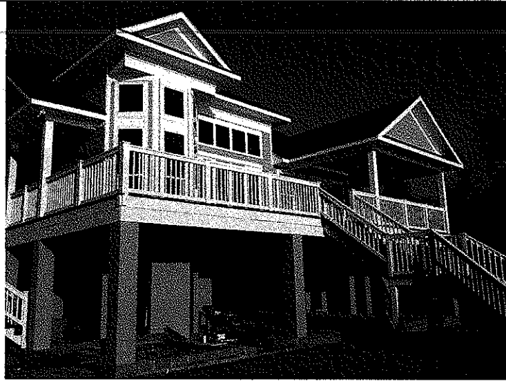
Rear View looking West 6/17/13, Lot 61, Riverwalk Subdivision
