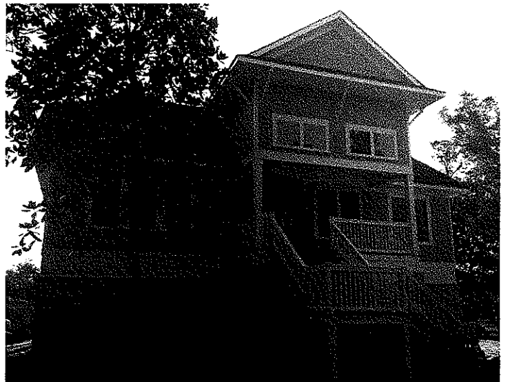
Front View, looking Northeast 6/17/13, Lot 61, Riverwalk Subdivision
