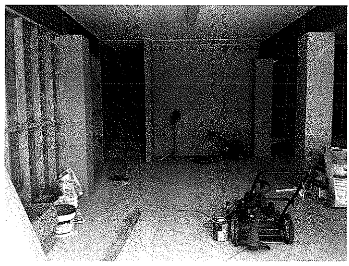
Side view of bottom enclosure in section A8, Lot 61, Riverwalk Subdivision 6/17/13
