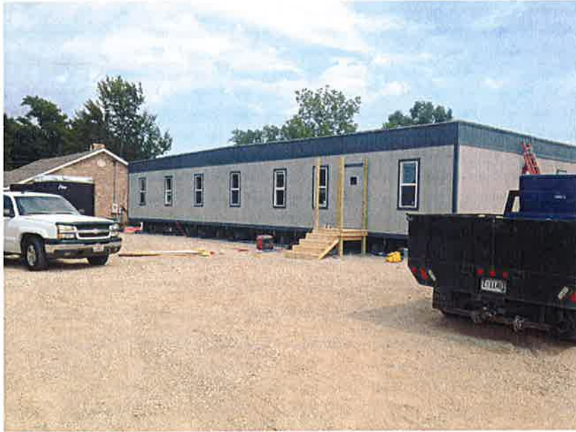
FRONT NORTH VIEW
