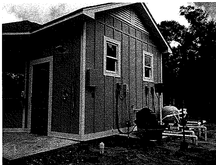
REAR VIEW OF POOL HOUSE. PICTURE TAKEN 8/20/2013
