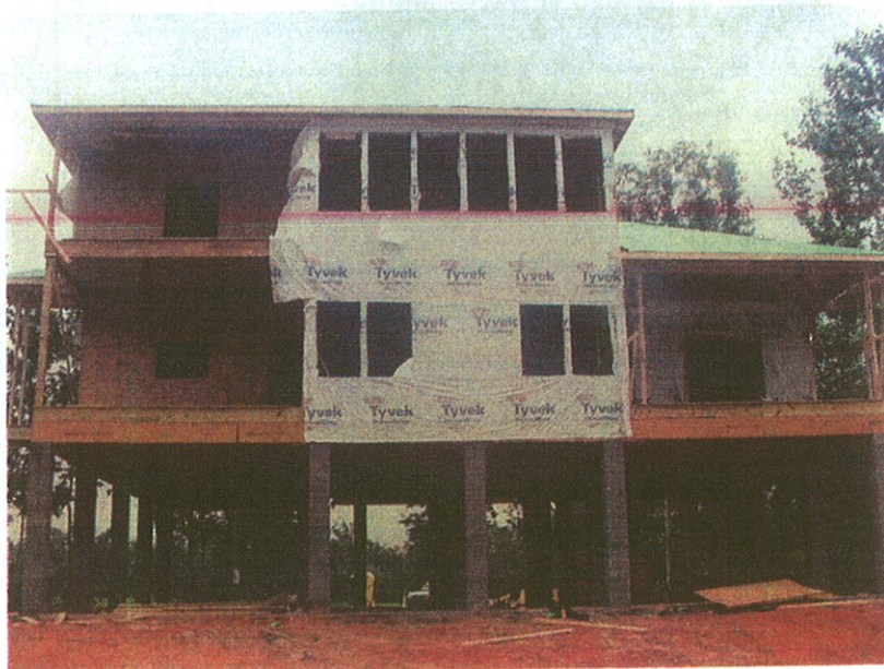
REAR VIEW OF RESIDENCE. PICTURE TAKEN 5/15/08.
