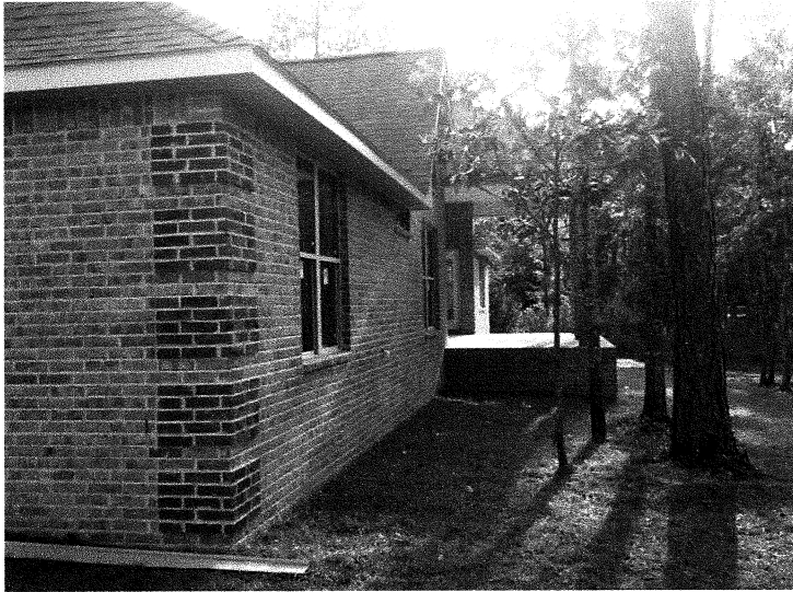
Northeast of the house looking Westerly along the northern side.
