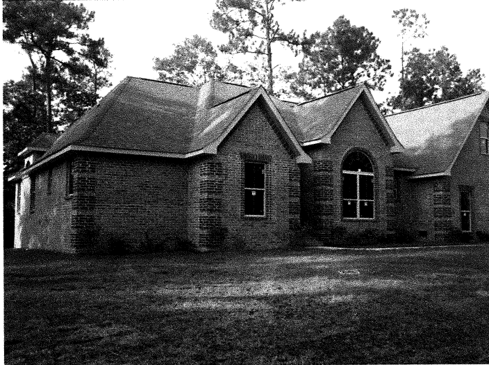
Southwest of the house looking Northerly along the Western edge.
