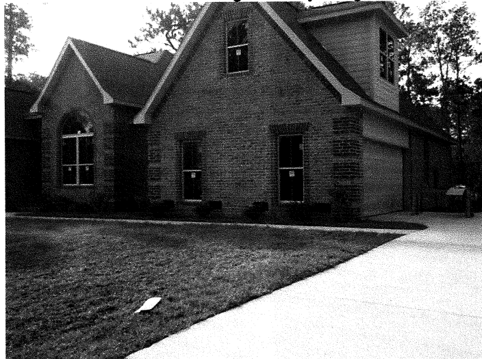
South of the house looking Northerly along the Eastern Edge side.
