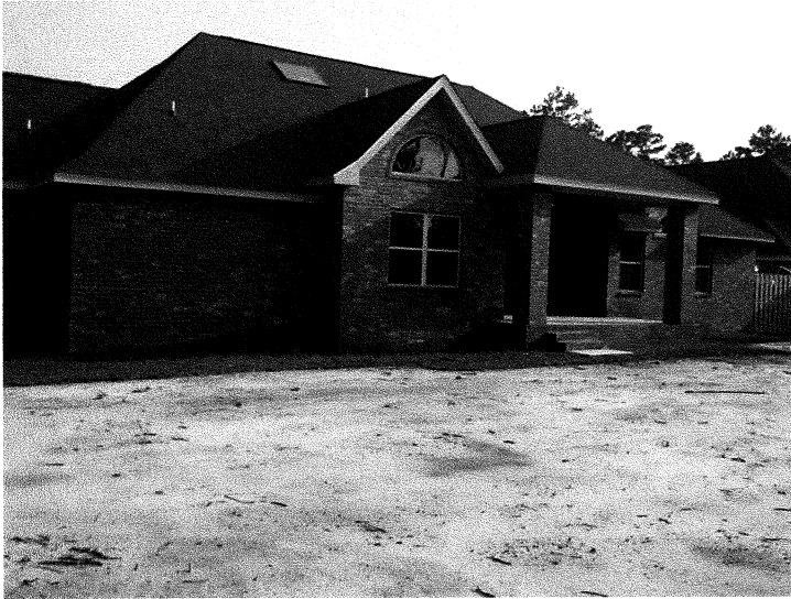
Northeast of the house looking Southwest.
