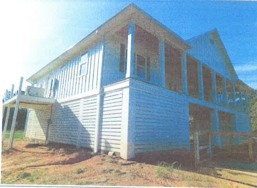
Photo Four Caption: REAR VIEW OF SITE
