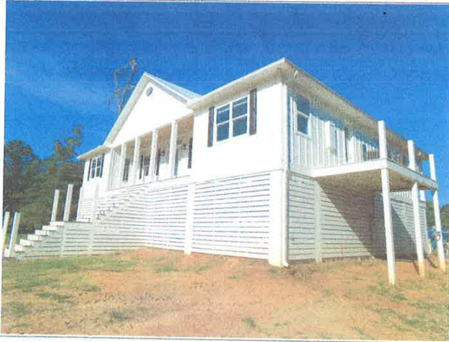
Photo Three Caption: FRONT VIEW OF SITE
